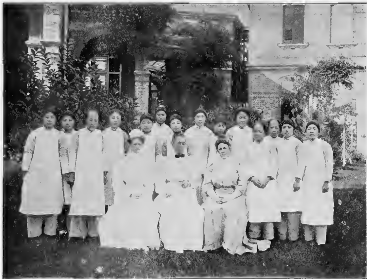
MARGARET WILLIAMSON HOSPITAL, WEST GATE.
